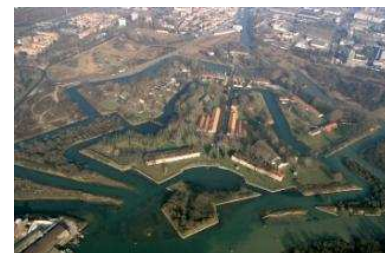
Aerial view of Forte Marghera
